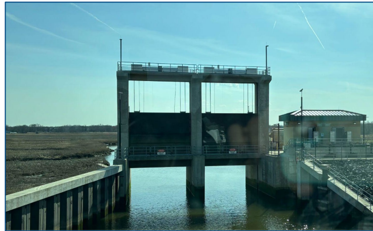
Port Monmouth Tide Gate and Pump Station. Source: J. Murray
